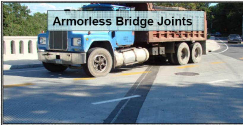
Ply-Krete® Joint Systems are poured in place to existing conditions providing extended service life at economical costs. It's ideal for bridges, parking decks, and commercial structures.
