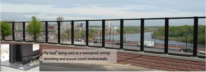
The Ply-Seal® Joint System consists of Ply-Seal®, a waterproof joint seal, and a two-part industrial adhesive that will bond to most any substrate to provide a flexible waterproof joint system. Ply-Seal<sup>®</sup> can be color matched to adjacent substrates in standard colors: back, gray, and beige.
