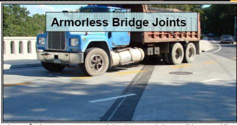
Ply-Krete<sup>®</sup> Joint Systems are poured in place to existing conditions. Providing extended service life at economical costs, it's ideal for bridges, parking decks, and commercial structures.
